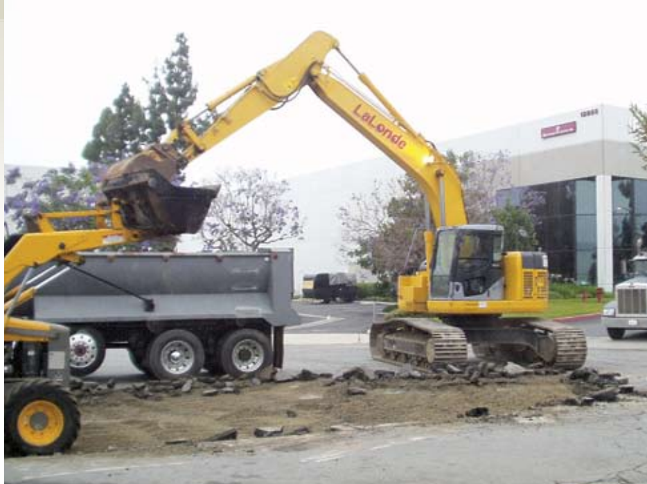
LaLonde Equipment Rental specializes in operated equipment rentals, providing both the machine and skilled personnel to operate it. Here, a LaLonde Equipment operator uses a Komatsu PC308USLC-3 excavator to remove part of an asphalt roadway for a customer.
