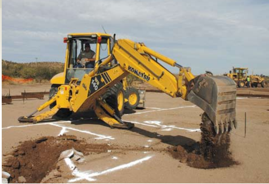
Using a Komatsu WB140-2 backhoe loader, Owner Mickey Dickson digs utility lines at a housing development in Tubac, Ariz.
