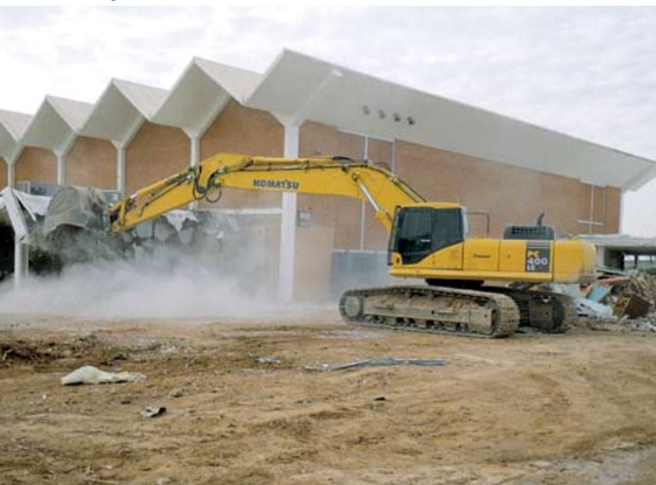
A Dickens Quality Demolition operator uses the company’s PC400LC-7 to take down a building in Phoenix.
