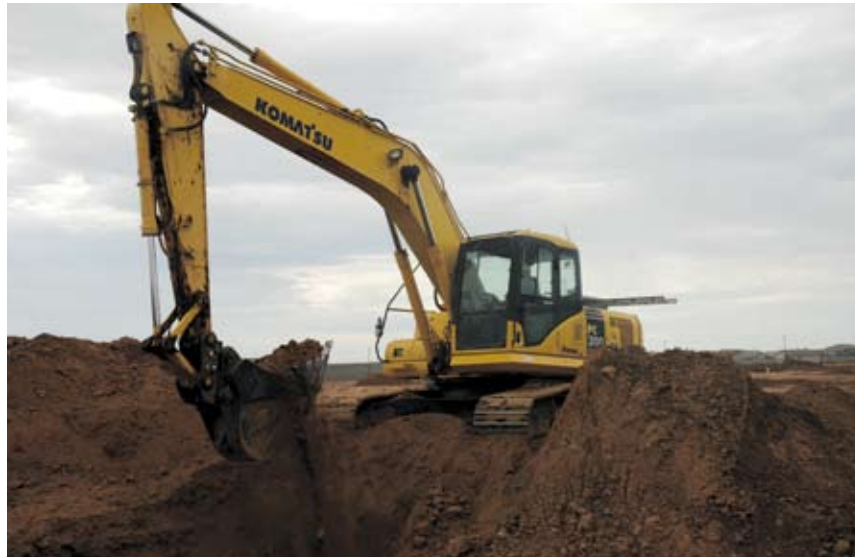
A D&A Pipelines operator uses a Komatsu PC200LC-7 to dig a utility trench at a housing development in Phoenix.
