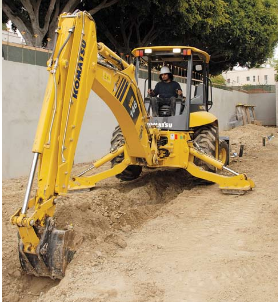
Using a Komatsu WB146-5 backhoe loader, Foreman Jesus Rodriguez Jr. digs a utility trench at the site of the new Rampart Police Station in downtown Los Angeles. "We use the WB146 for shallower digs, but we can also backfill with it and put a wheel on it for compaction," said Owner Jesus Rodriguez. "It helps us in tight spaces too, where we can't fit a bigger machine."
