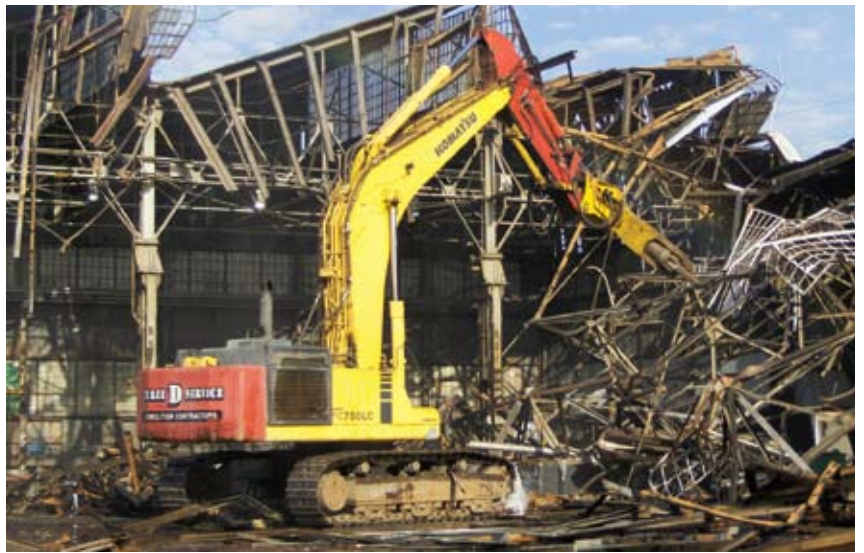
A Three D Service operator processes scrap-iron materials, using a Komatsu PC750 excavator, prior to loading them out.
