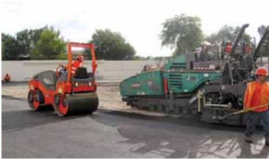
Road Machinery added asphalt paving to much of the area surrounding its new Gilbert branch. S&S Paving did much of the work using Road Machinery's HAMM and Vögele paving products.
