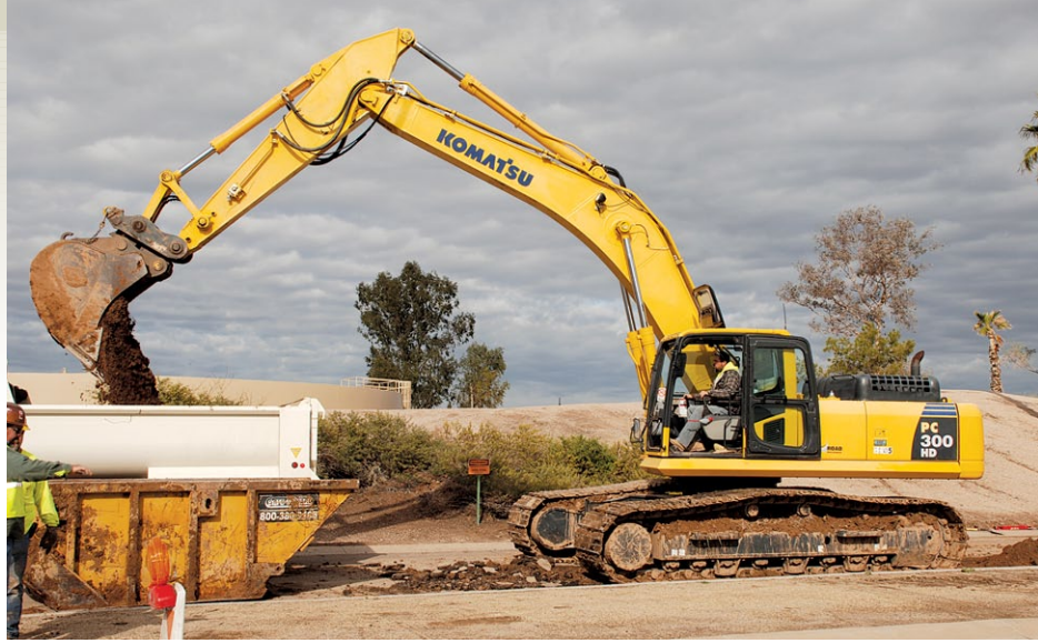
An Arizona State Utilities operator uses a Komatsu PC300HD-8 to load a truck at a water-line installation project for the city of Chandler. "It has a little more beef underneath it, so it's sturdier in the deeper digs," said General Manager Wayne Dawson of the heavy-duty excavator.
