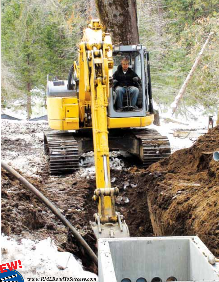
Foreman Russell Allison digs a trench for installation of new power lines using a Komatsu PC128UU excavator.
