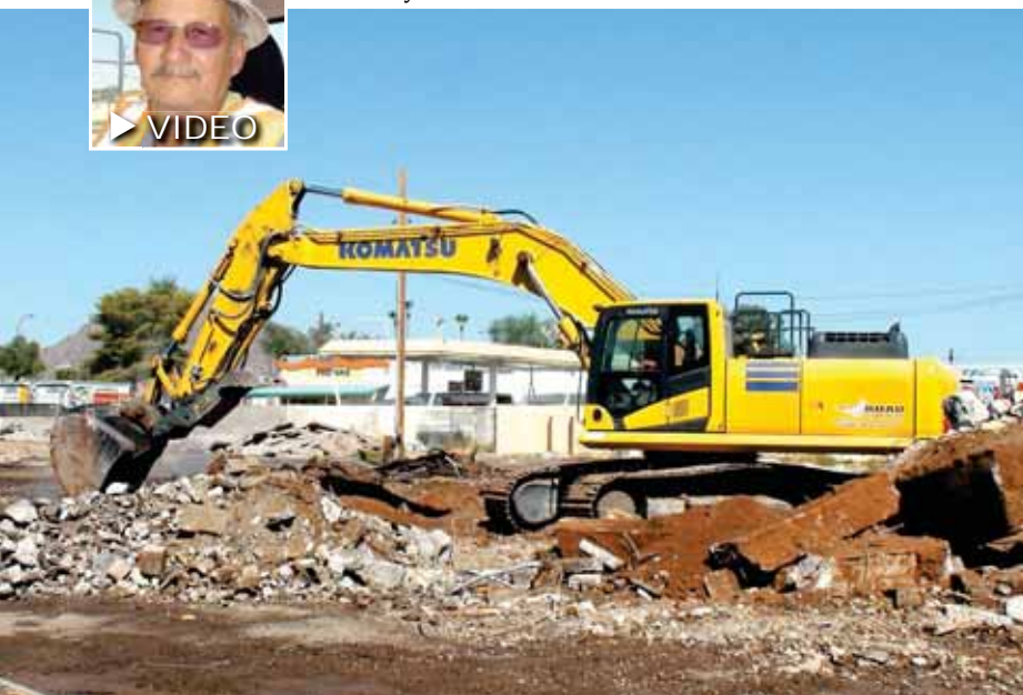
Operator Rick Bailey removes paving with a Komatsu PC360LC-10 excavator that Arizona Specialty Demolition rented from Road Machinery LLC.
