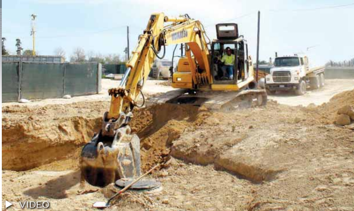
Ground Breakers Construction uses a Komatsu PC210LC-10 excavator equipped with a Topcon GPS system to dig utility trenches.
